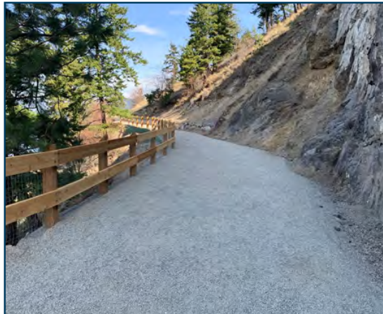
3. Paul’s Tomb – Widened for Improved Access
