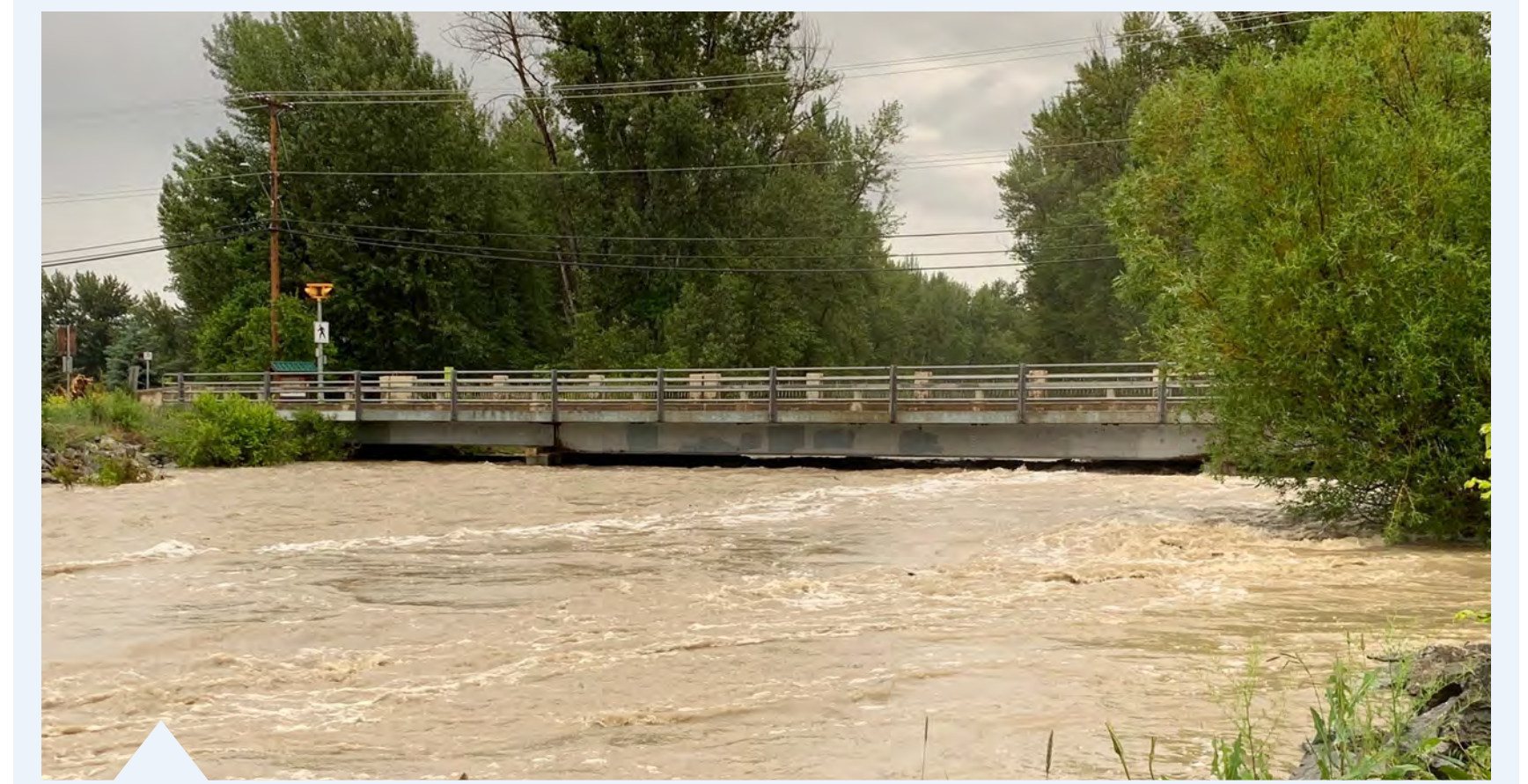
Low bridge height and concrete pile, in-stream
