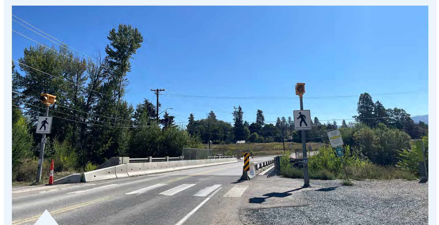
At-grade Greenway trail crossing with pedestrian flashers
