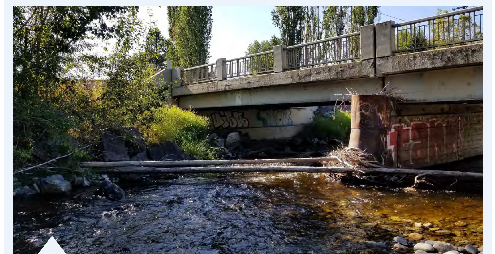
Concrete pile creates barrier for in-stream debris
